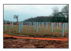
Construction well under way with the majority of posts to support 55,000 panels in place.
